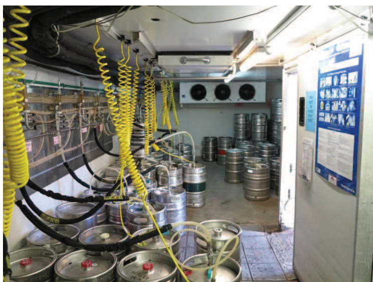
Figure 4.9: Photo showing the width of the interior of the cellar. Photo taken looking north, C&L 2014.
