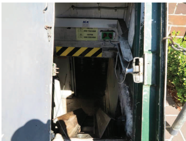
Figure 4.8: Photo showing the access to the cellar from Harris Street and an indication of the depth of the cellar. Photo taken looking west, C&L 2014.
