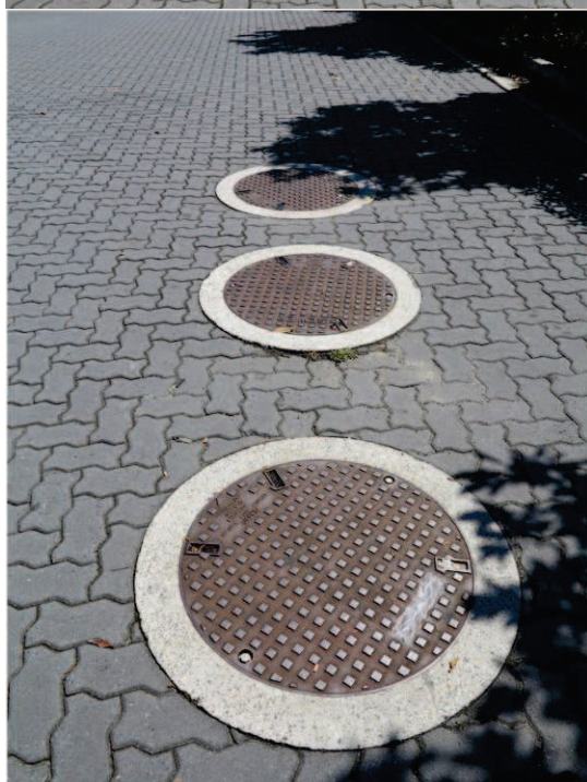
Figure 4.11: Three pit covers marked 'sewer' on the eastern side of the carpark. There was also a pit cover marked 'electrical' in the same area. All these services are likely to be deep impacts. Photo taken looking north, C&L 2014.
