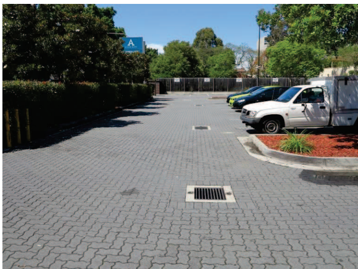
Figure 4.10: Photo showing the pits associated with the eastern-most stormwater in the carpark. Photo taken looking south, C&L 2014.
